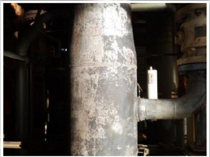
*DRY ICE CLEANING REMOVES HEAVY CORROSION AND DEFECTIVE COATINGS FROM PIPEWORK AND ALLOWS FOR MINIMAL DISASSEMBLY, NO DRYING TIME, REDUCED ENCAPSULATION AND WASTE DISPOSAL, WHICH OPTIMIZES THE OVERALL PROJECT TIME.*
